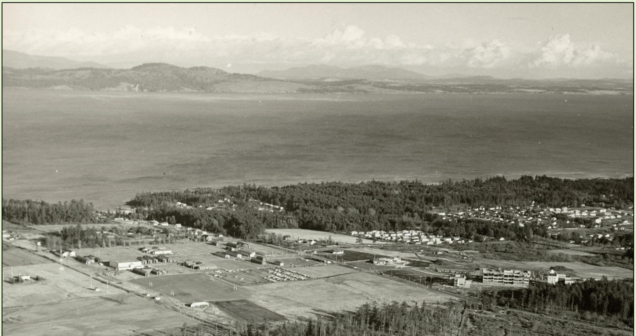
Aerial view of Gordon Head, showing University of Victoria campus under construction at right and Gordon Head Army Camp left of centre, 1960s (detail of 1995-004-011)
